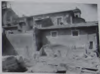
Fig. 216. W. BURNETT, SOUTH WALL FOUND, DEMONSTRATION OF BUILDING PHASES, 1938
